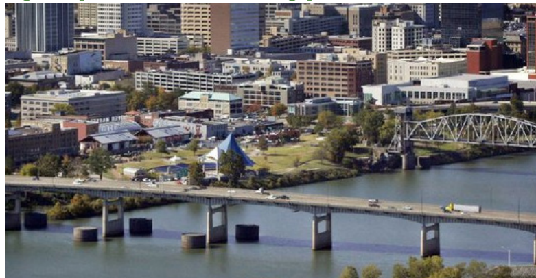
Figure 8 [I-30 Arkansas River Bridge]
