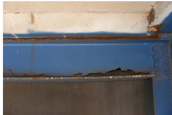
Figure 10 [Beam Corrosion]
